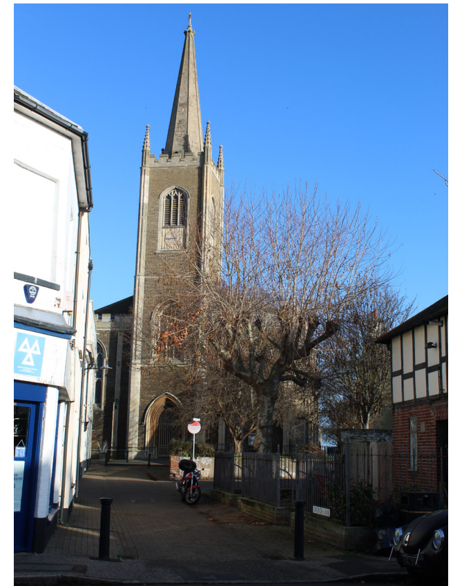
Figure 38 View along Church Lane
