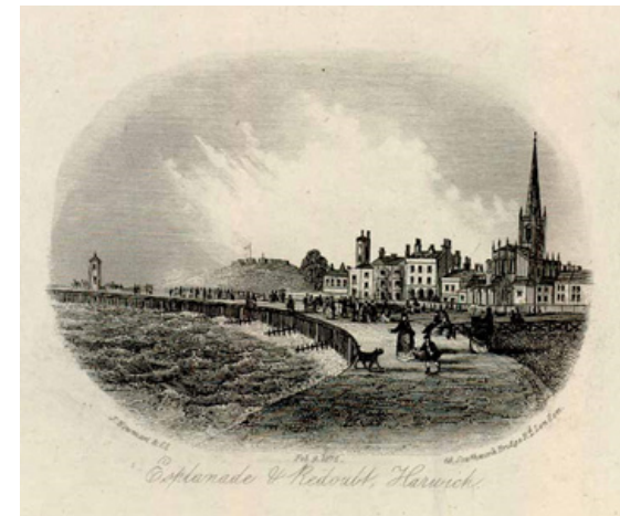
Figure 8 Esplanade and Redoubt, Harwich 1876 (ERO X172-19 Imp 120-1-3)
