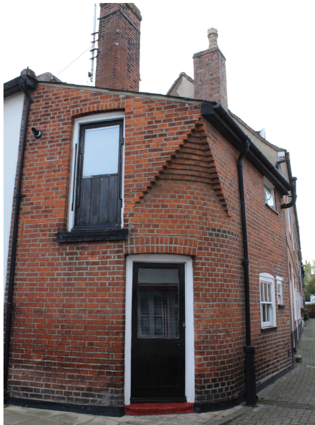
Figure 37 Building detail on George Street
